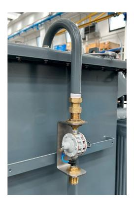
3. Wrap the teflon on the lower connector of the device. Screw the dehydrating Breather on the connector.
