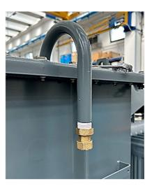
2. Screw the device to the fitting previously mounted on the transformer tube. Be careful to position the gasket provided for sealing between the two fittings
